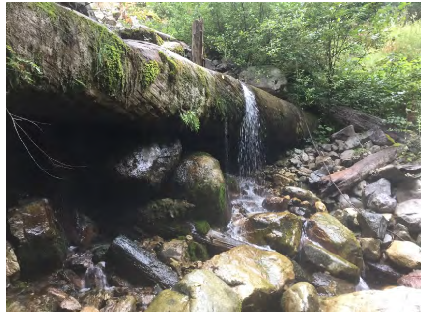
Log retaining fill anchored in middle (approx) and left bank
