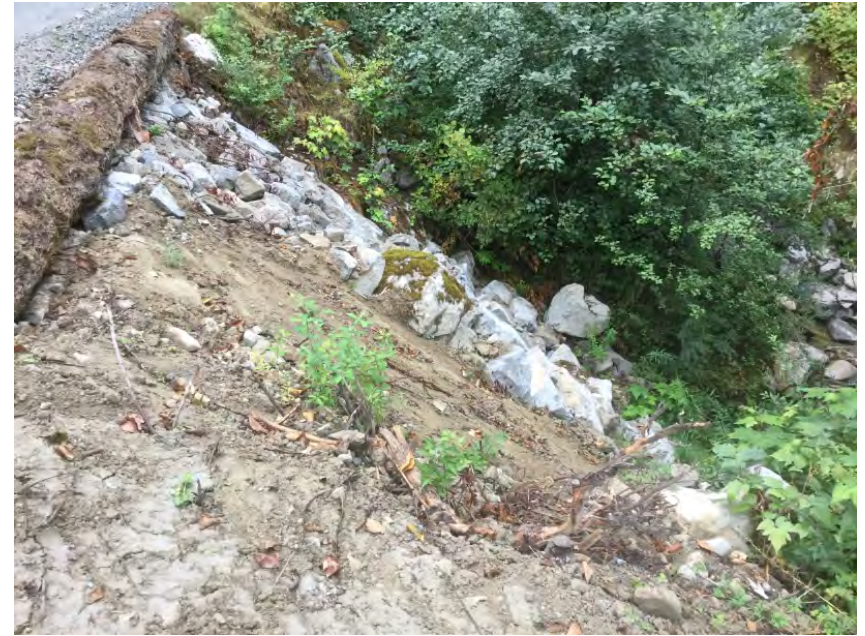
Downstream right approach fill slope repair
