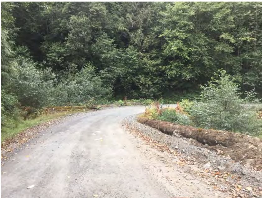
Approach from Right Bank when facing downstream
